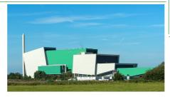
It is not just any old incinerator. It is state of the art. It feeds on 210,000 tons of domestic waste (i.e non-recyclable) a year, which is burnt at a temperature of 850 degC. The ash is processed to remove metals, both ferrous and non-ferrous, which can be recycled; what remains is passed on as industrial aggregate. The gases are 'scrubbed' using lime and activated carbon, and then passed through filters to remove particulates. What comes out of the chimney is mainly steam and carbon dioxide.
